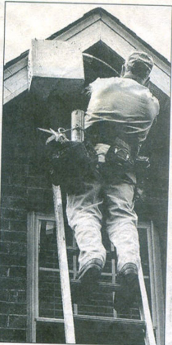
CRAIG CUNNINGHAM/DAILY MAIL To clear bats from an attic, Braley relies on a special metal trap that he bolts over the tiny holes bats use as entrances and exits. Braley began removing animals from homes after the state started licensing eviction specialists six years ago.
